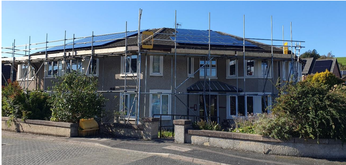
Panels being installed at the Lapwing Housing Co-operative in Halton
